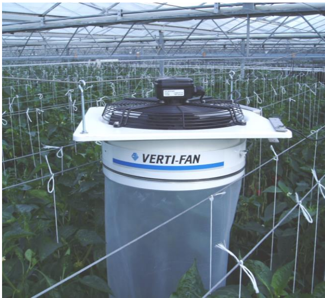
Picture 2 Verti-Fan with cable installation
